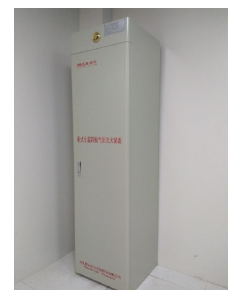
气体消防柜 Gas fire control cabinet
